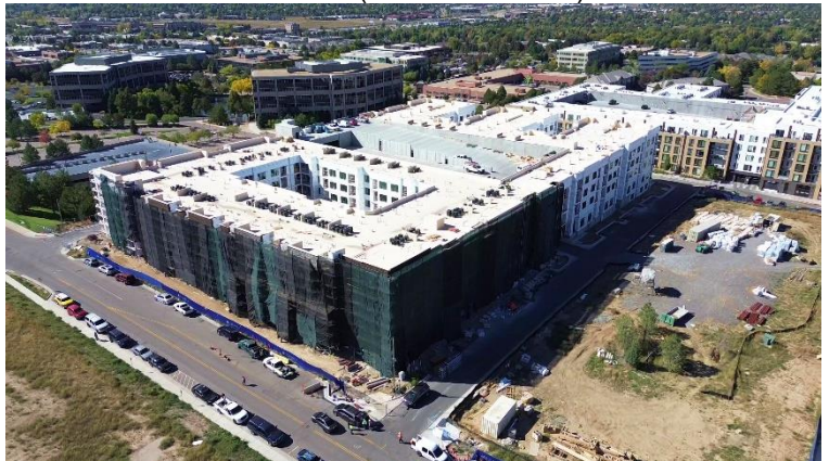
Parcels 6 & 7 (View: Southwest)
