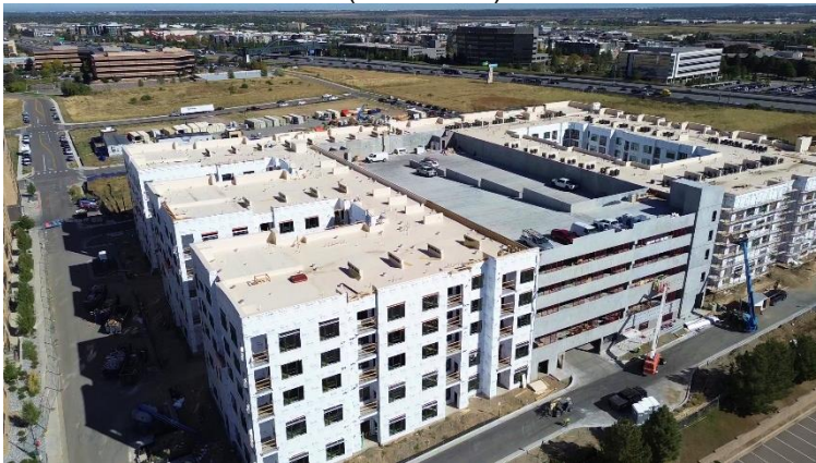
Parcels 6 & 7 (View: Northeast)
