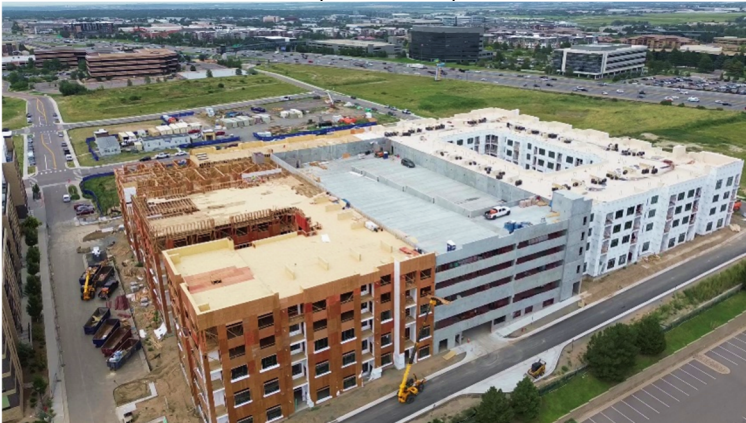
Parcels 6 & 7 (View: Northeast)
