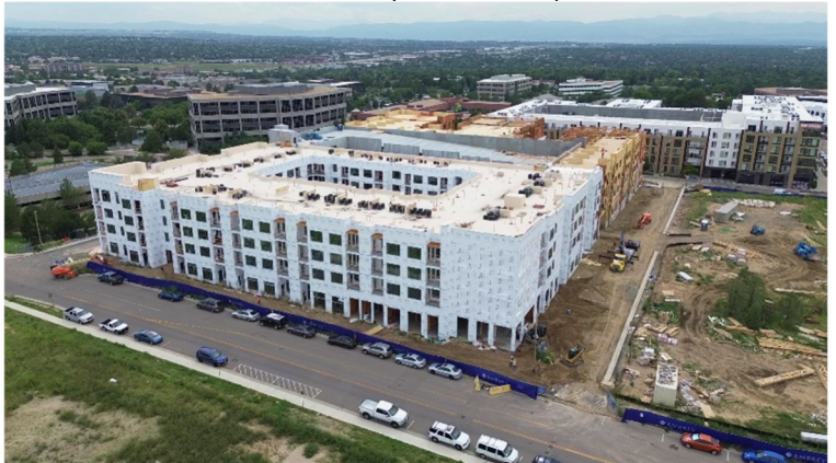
Parcels 6 & 7 (View: Southwest)
