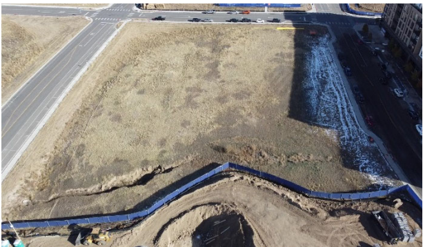
Parcel 9 (View: East)
