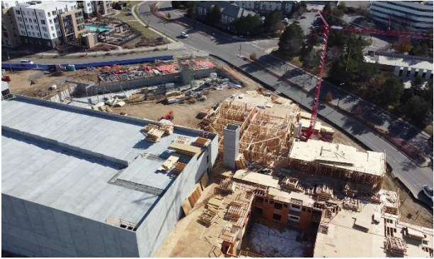
Parcel 8 (View: South)
