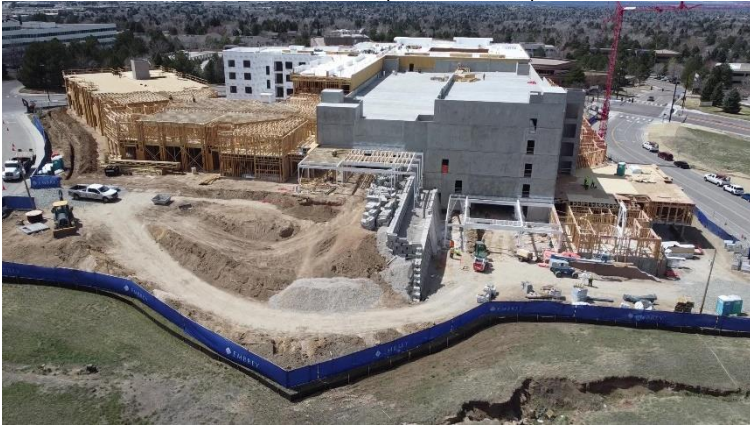
Parcel 8 (View: West)
