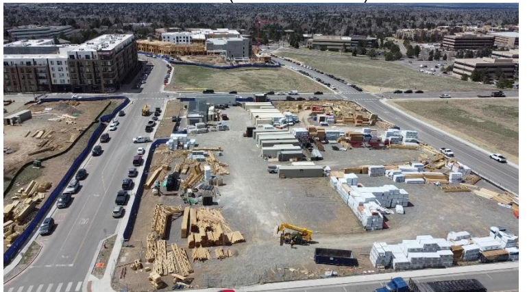
Parcel 11 (View: West)
