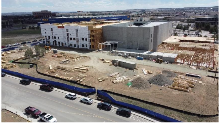
Parcels 6 & 7 (View: Southeast)
