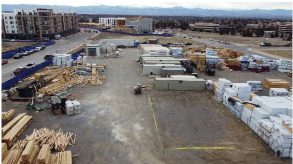
Parcel 11 (View: West)
