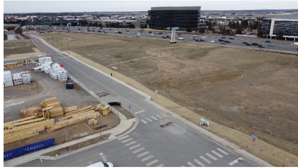
Parcels 1 & 2 (View: Southeast)
