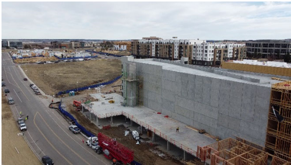
Parcels 8 & 9 (View: Northeast)
