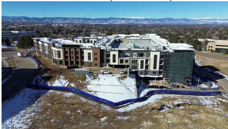
Parcel 8 (View: West)
