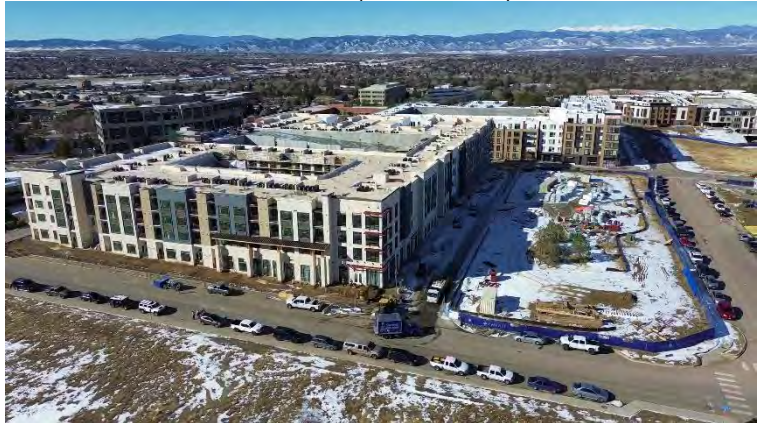
Parcels 6 & 7 (View: Southwest)
