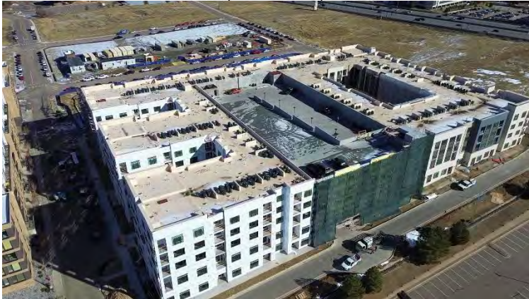
Parcels 6 & 7 (View: Northeast)
