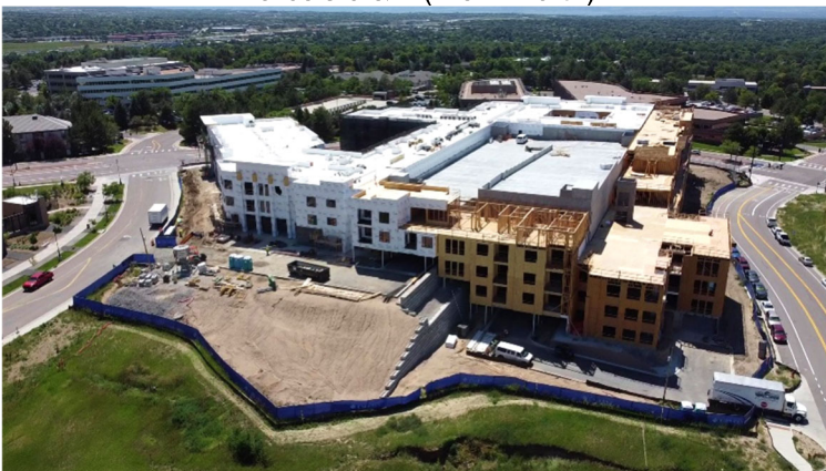
Parcel 8 (View: West)
