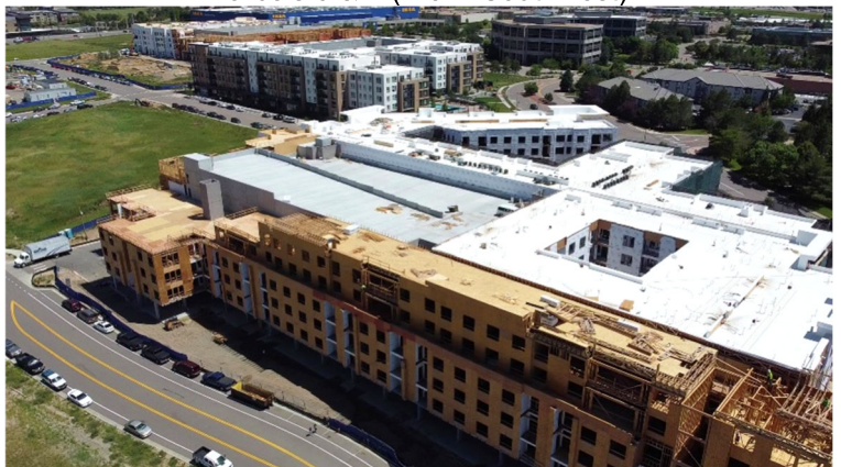
Parcel 8 (View: Southeast)
