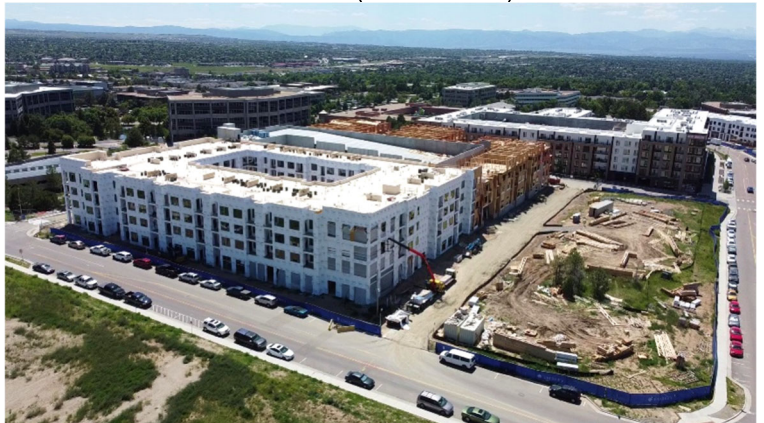
Parcels 6 & 7 (View: Southwest)
