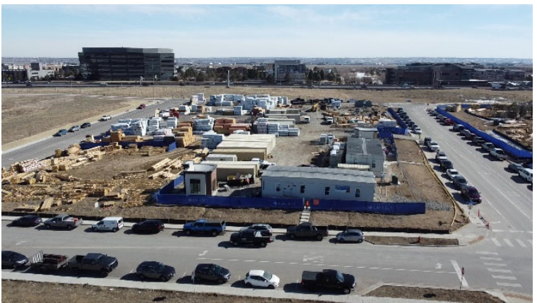
Parcel 11 (View: East)
