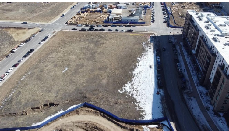
Parcel 9 (View: East)
