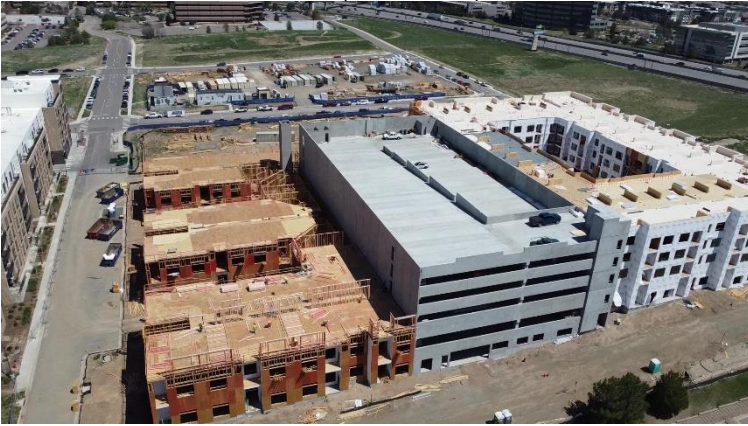
Parcels 6 & 7 (View: Northeast)
