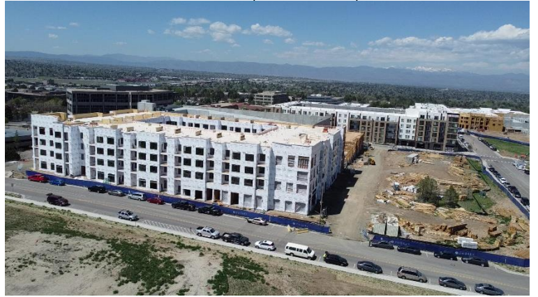
Parcels 6 & 7 (View: Southwest)
