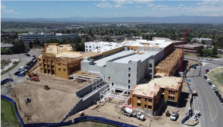
Parcel 8 (View: West)
