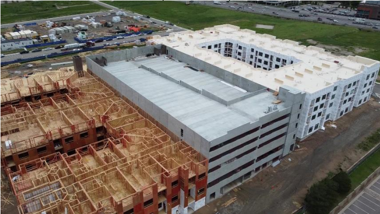
Parcels 6 & 7 (View: Northeast)
