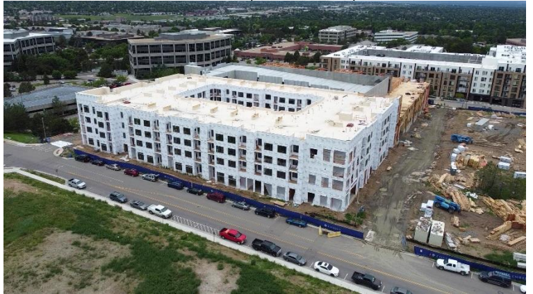
Parcels 6 & 7 (View: Southwest)
